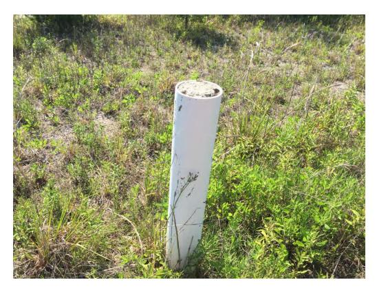
Figure 11 - View of concrete capped pvc pipe at abandoned processing facility
