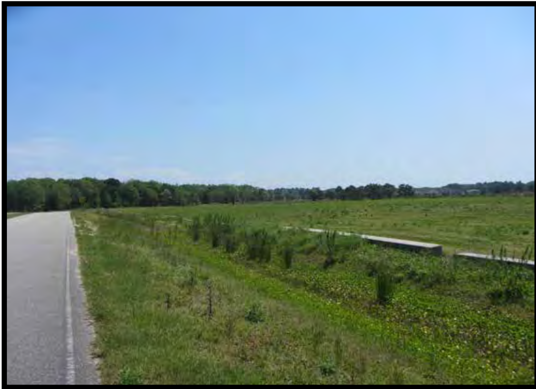
Photograph # 13: View along Sandridge Road Ext.
